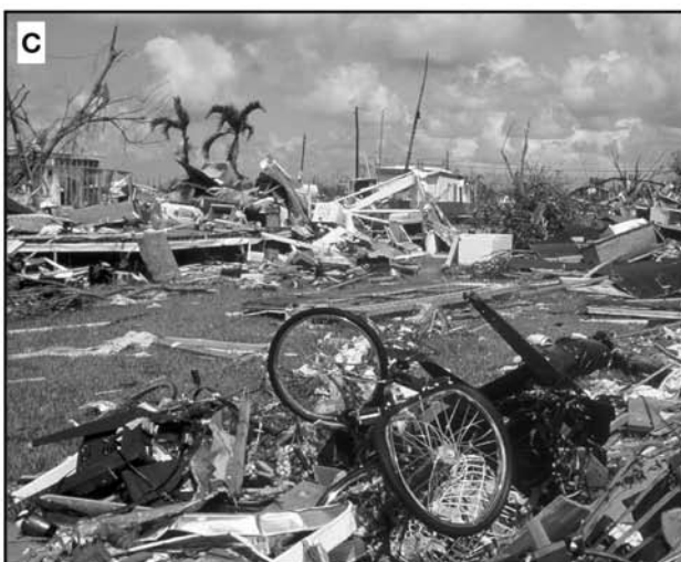
Destruction caused by Hurricane Georges in Florida
